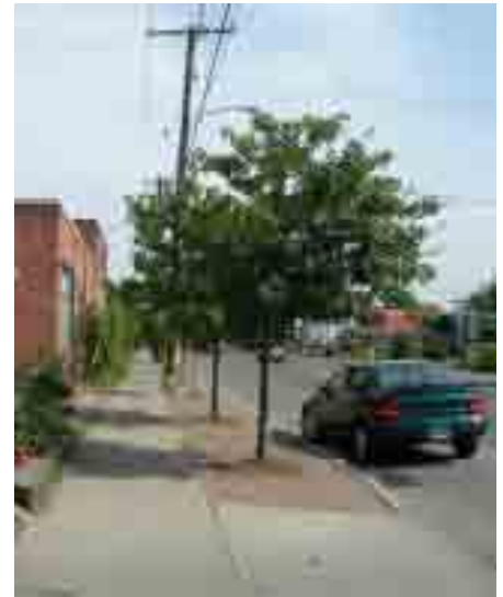
Fig. 1.24 Concrete unit pavers on a coarse sand setting bed on top of a continuous trench of CU-Structural Soil™ in Ithaca, NY
