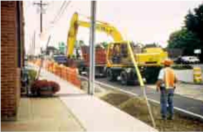
Fig.1.9 Installing CU-Structural Soil™ in Ithaca, NY in 1997
